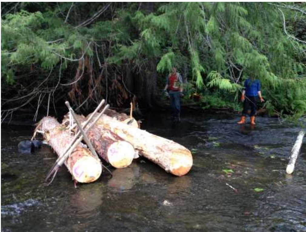
Photo 2. Logs staged in the Quinsam River ready to be moved into position.
