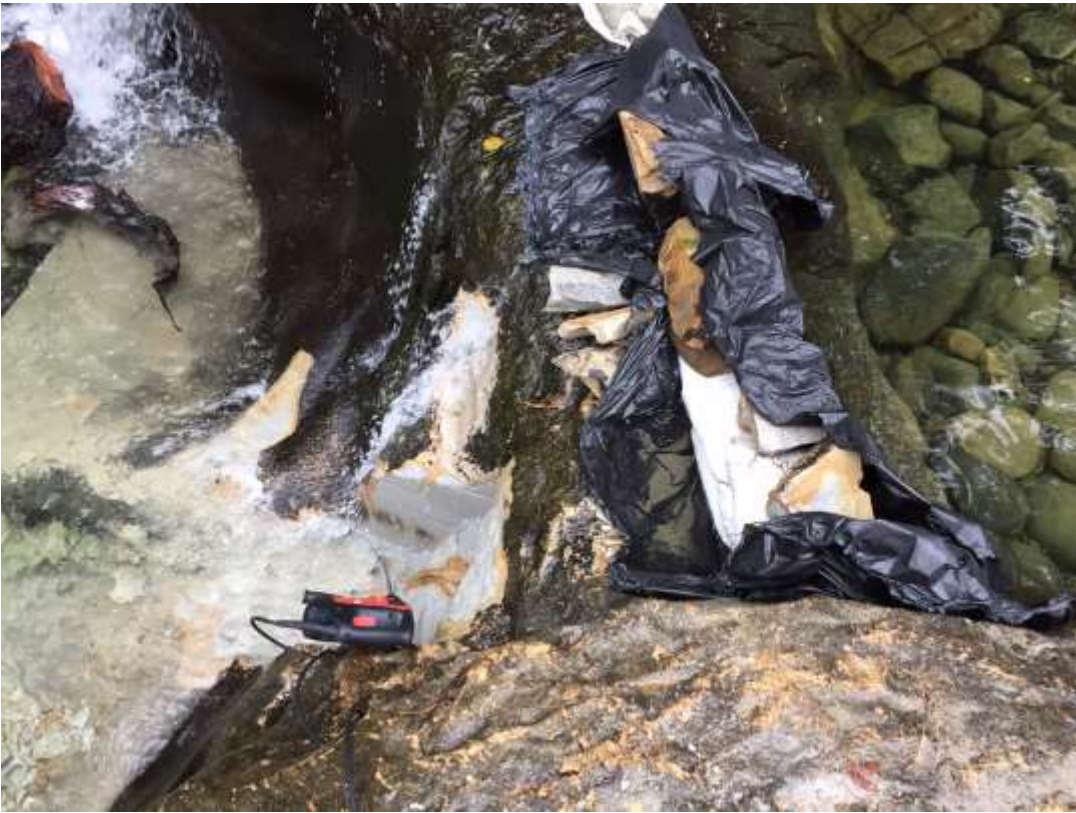
Photo 4. Plastic sheeting increased effectiveness of sandbag dams.
