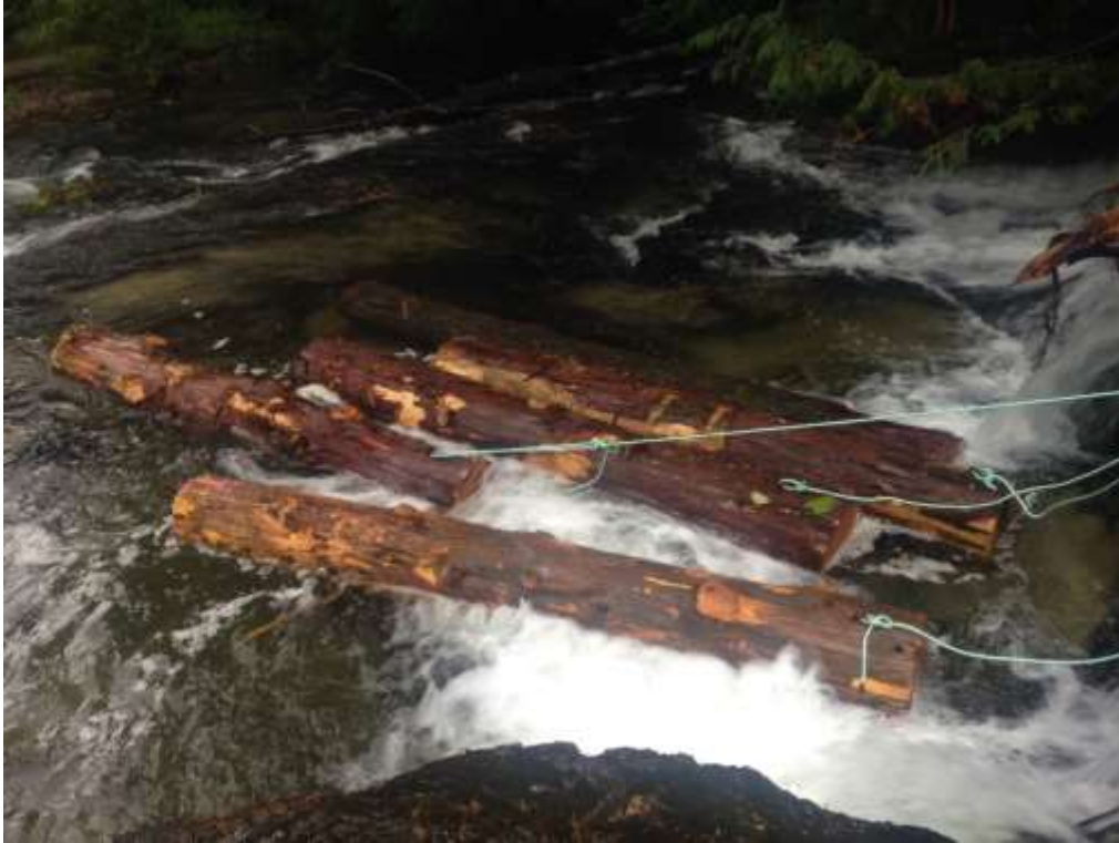
Photo 1. Logs staged in the Quinsam River tied to bedrock.
