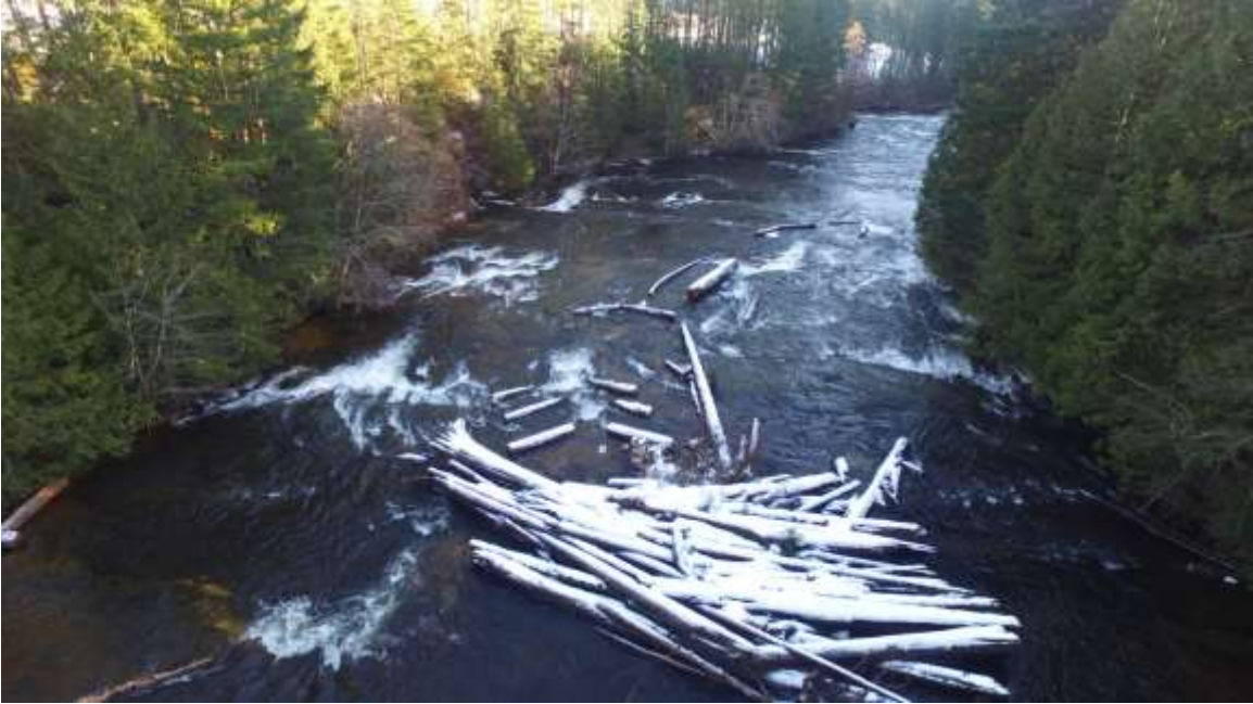
Photo 18. Aerial view of the upper site showing the effectiveness of the anchored logs at confining and redirecting flow.
