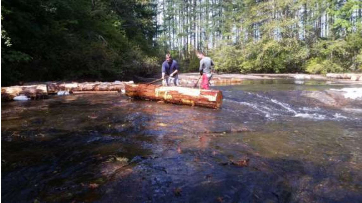
Photo 6. Logs being moved into position using Pee Vees.
